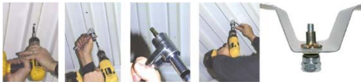
Step 1 Step 2 Step 3 Step 4 Completed Installation
